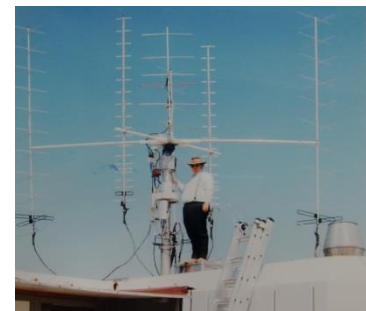
▲ GSOC's VHF antenna on the rooftop for voice transmissions with MIR (courtesy of George Hiendlmeier, GSOC).
